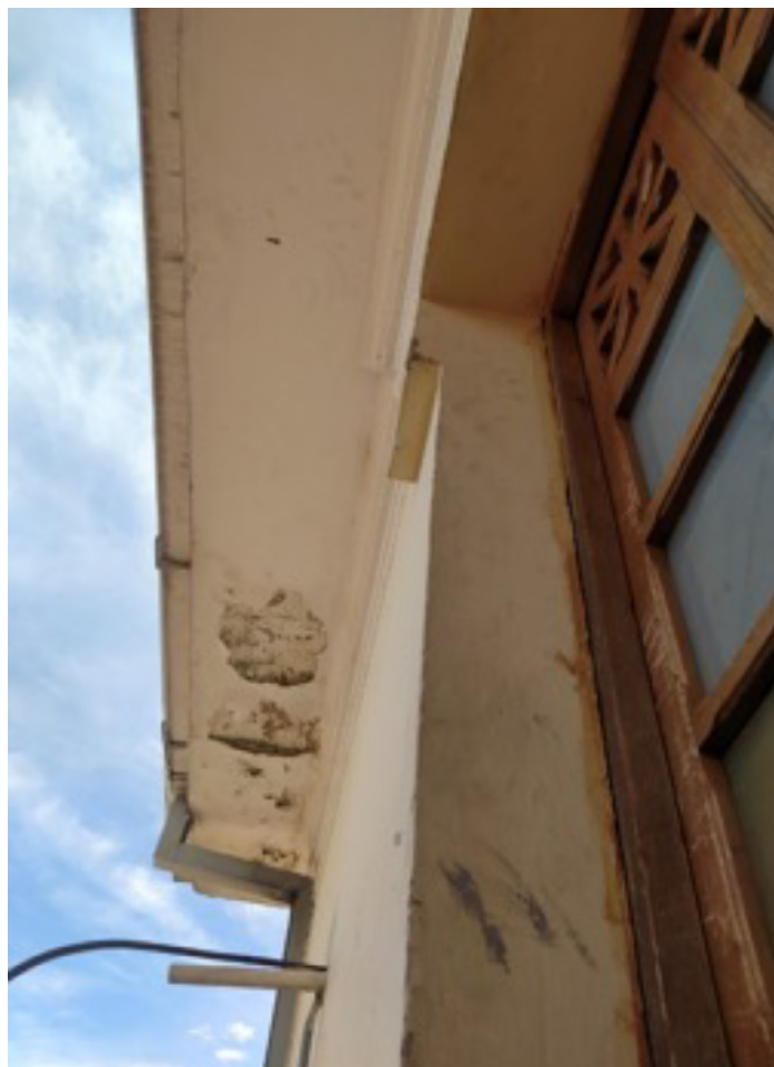
Figure 10. Moisture Due to Atmospheric Conditions
