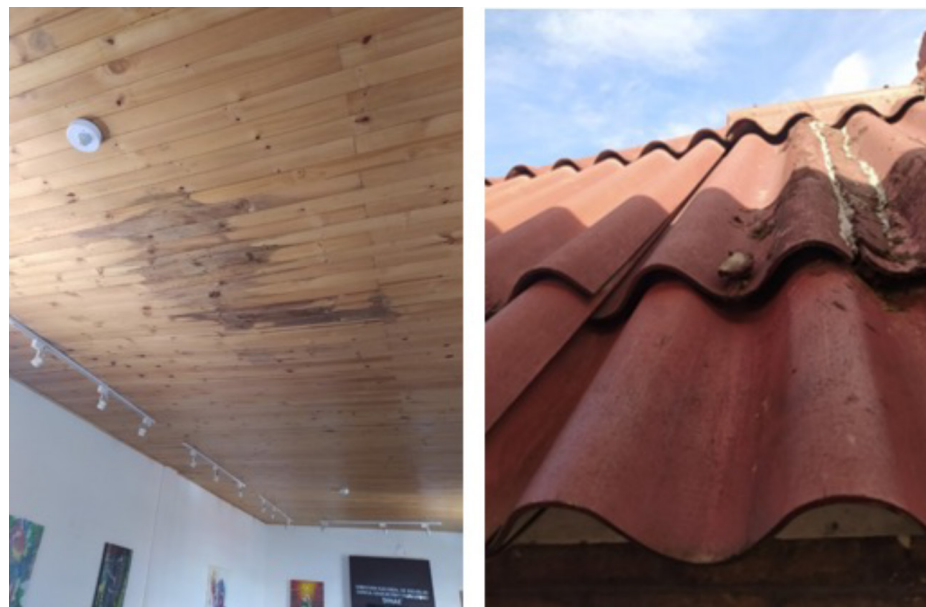
Figure 8. Moisture Due to Absorption
