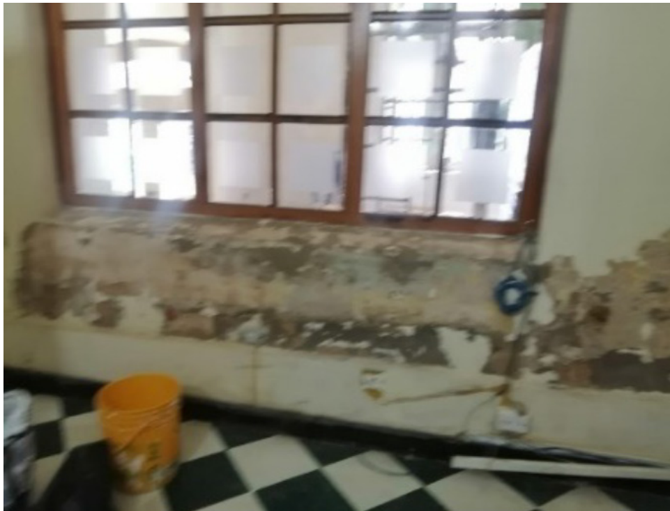
Figure 7. Capillary Moisture
